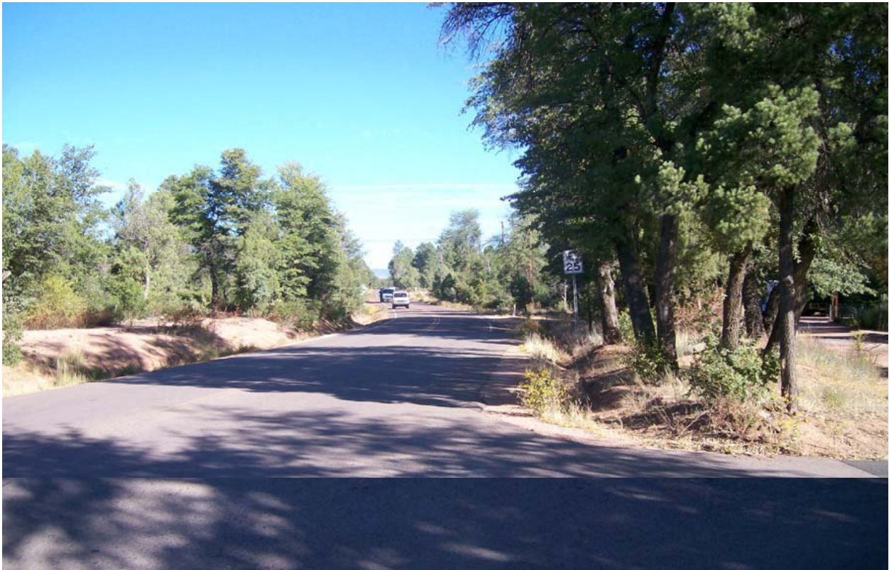
McLane Road just North of Airport Road
