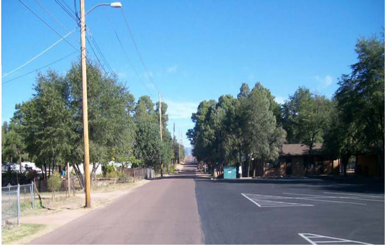
Colcord Road just North of Bonita Street
