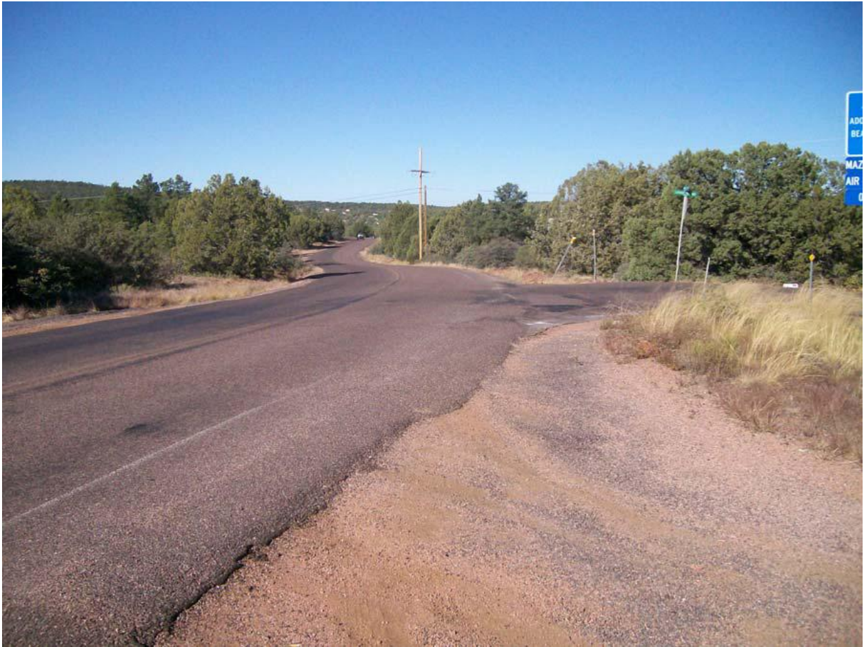
Airport Road at Earhart Parkway
