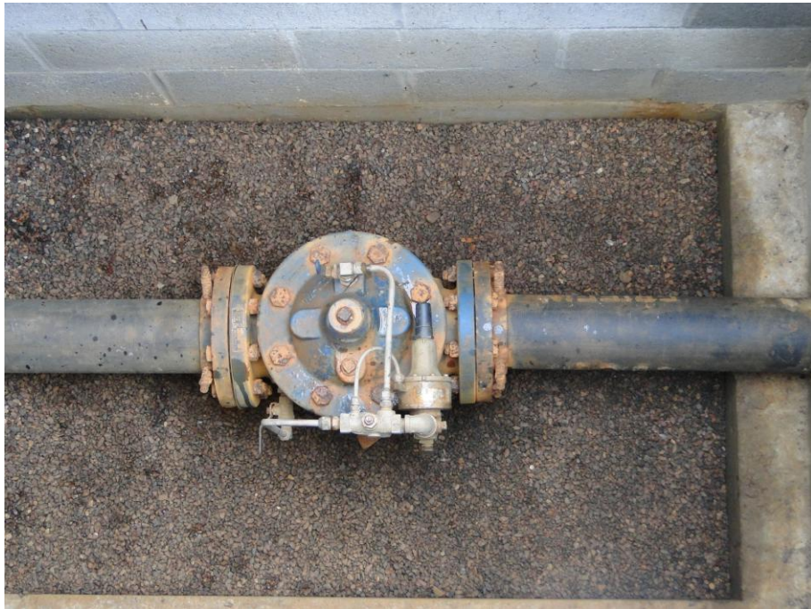
An existing PBV near Graham Ranch Trail
