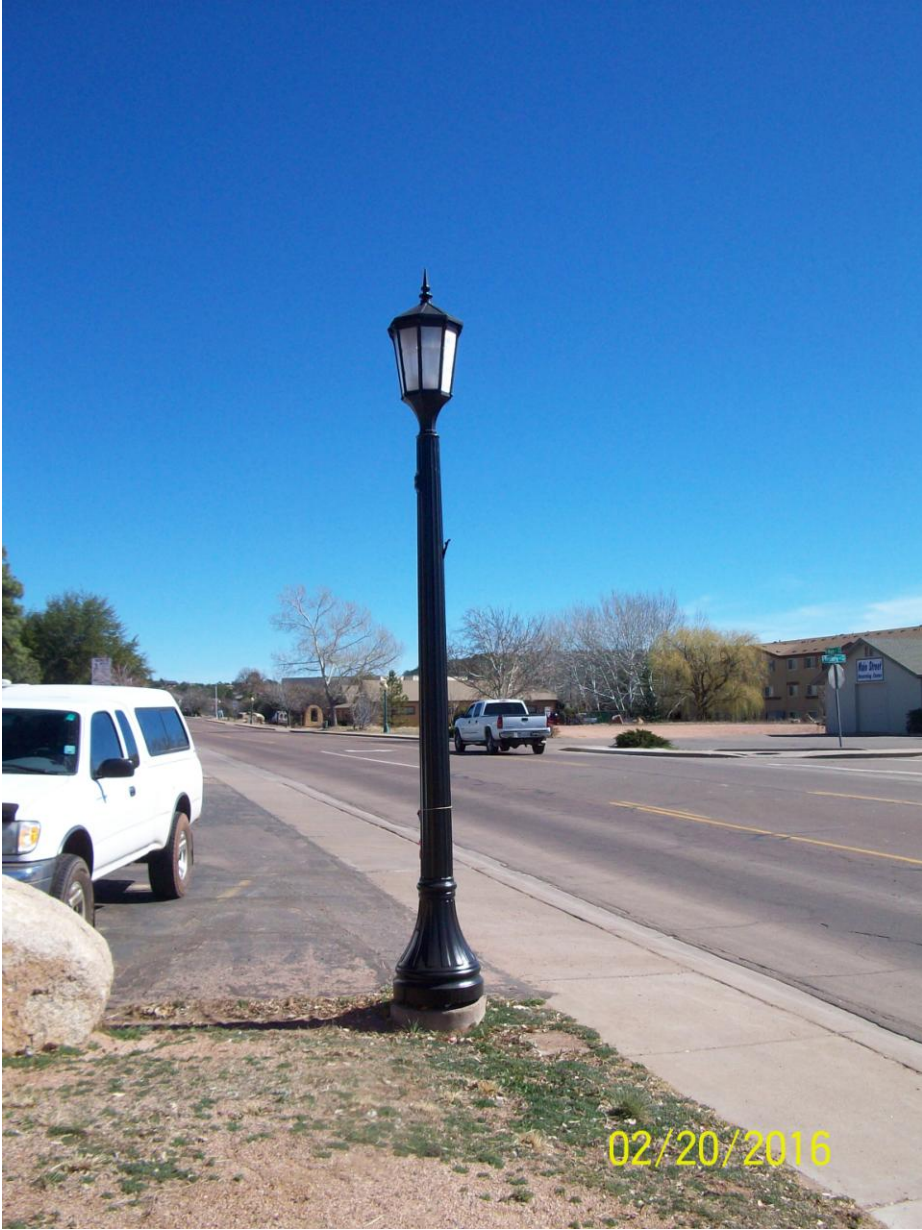
New Replacement LED lights
