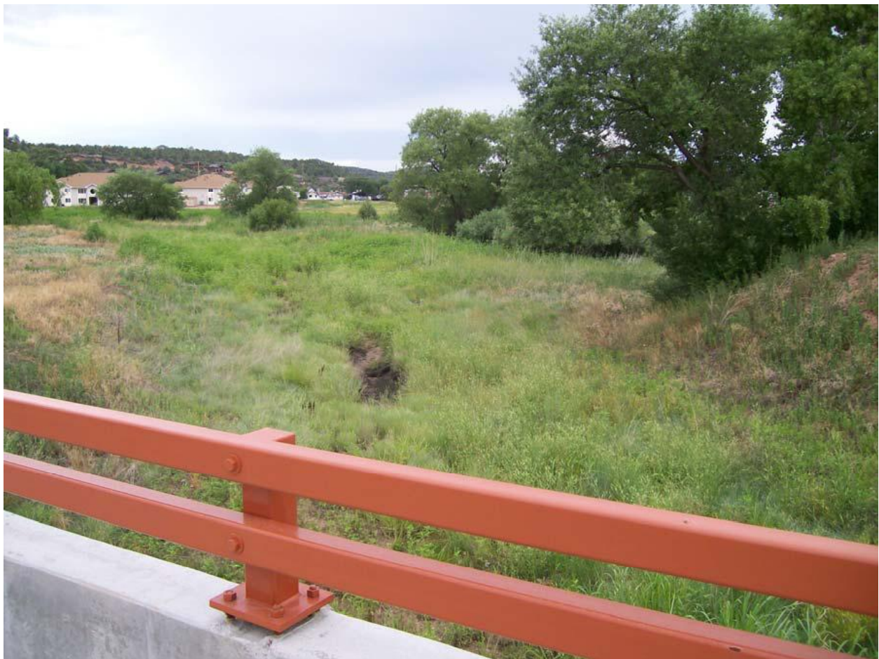
American Gulch looking west from Westerly Road
