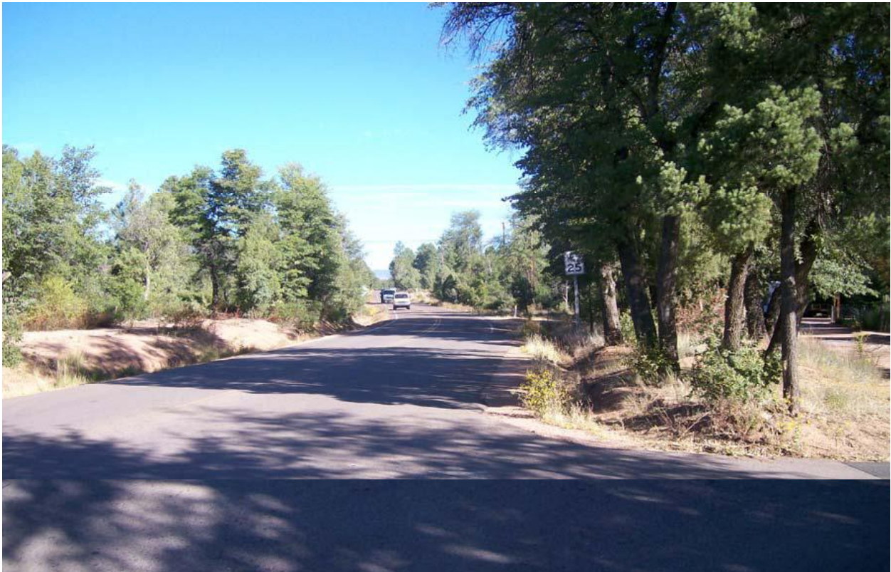
McLane Road just North of Airport Road
