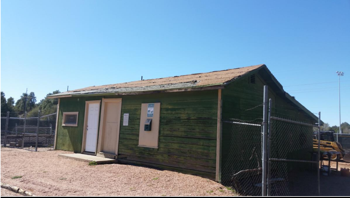
Existing Parks Maintenance shed
