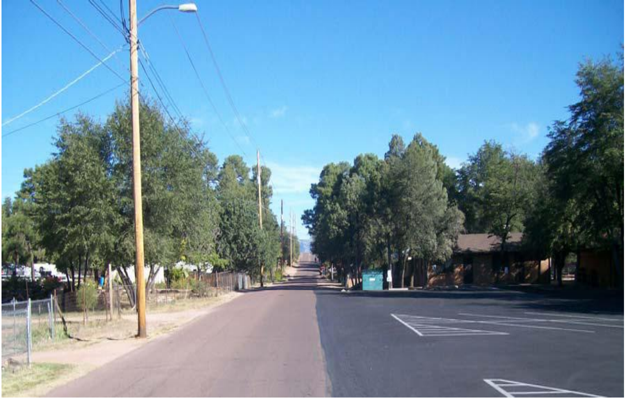
Colcord Road just North of Bonita Street
