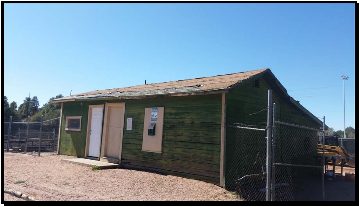
Existing Parks Maintenance shed.
