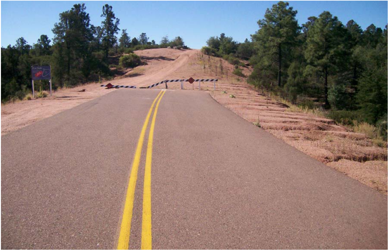
Rim Club Parkway Extension south of the Rim Golf Course Entrance
