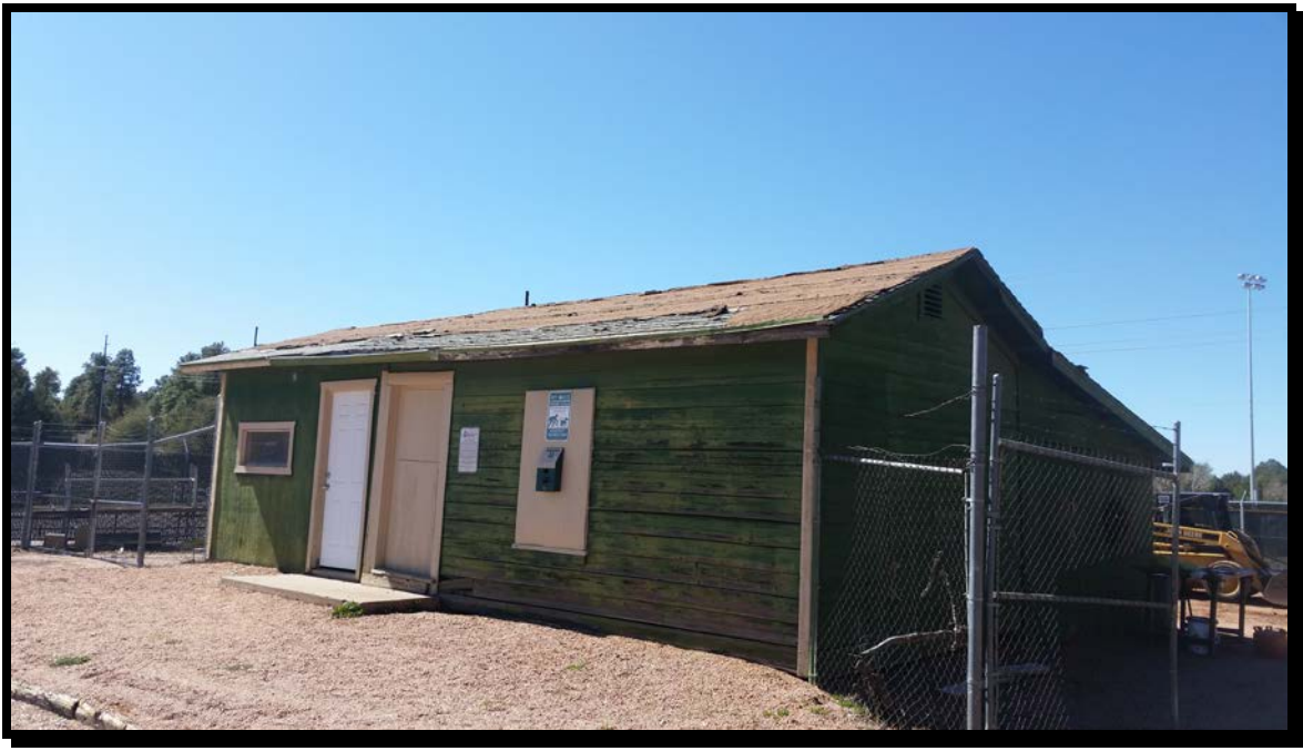
Existing Parks Maintenance shed.
