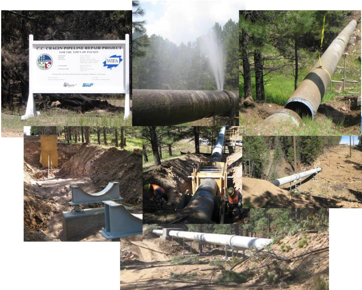
Cragin Pipeline Repairs 2009 –Courtesy PCL Contractors and SRP
