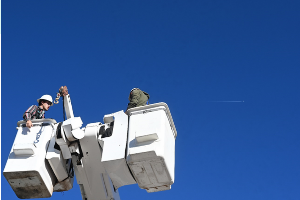
Jesse and KC prepare in the boom truck to handle and hang lighting and decoration for the Giant Sequoia on the south side of 260 near McDonald's.
