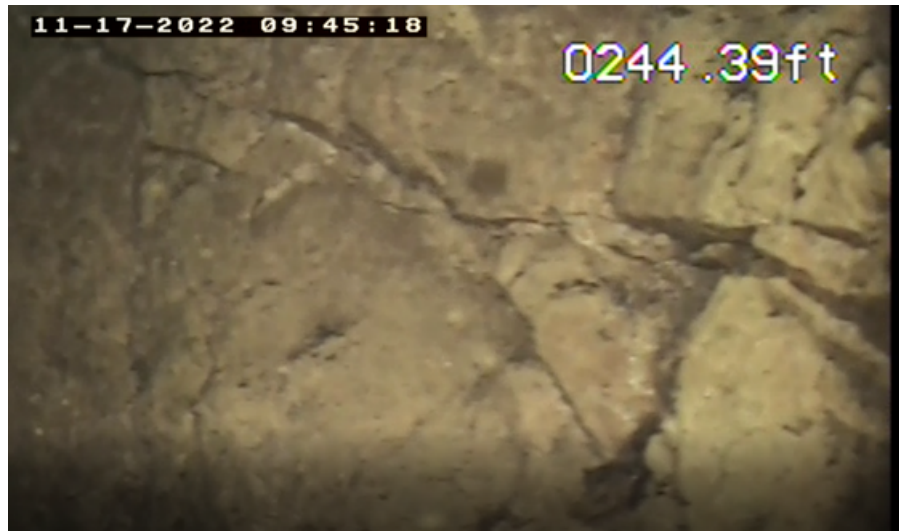
View of the bare aquifer wall showing the fractured nature of Payson's aquifer.
