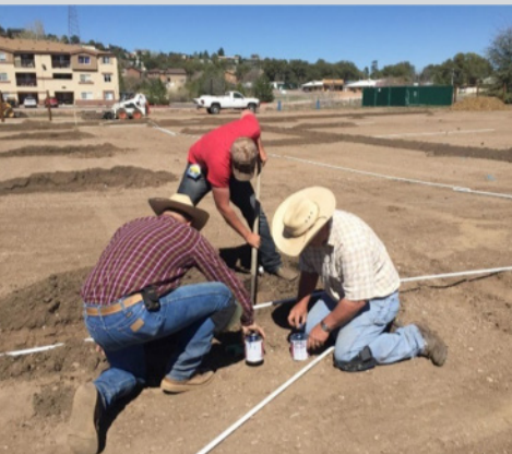
Installing Irrigation for Orchard.
